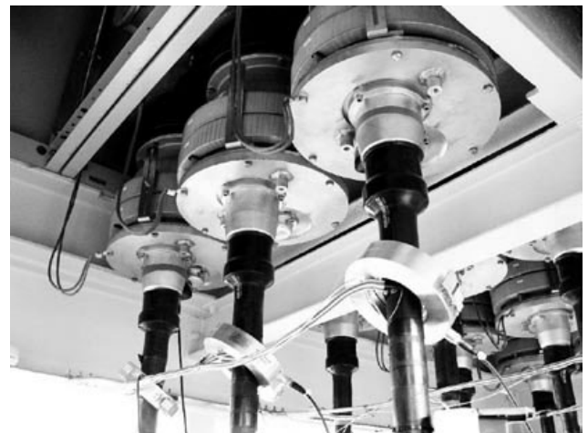
Figure 5: HF CTs installed on sheath earths of 33 kV cable
